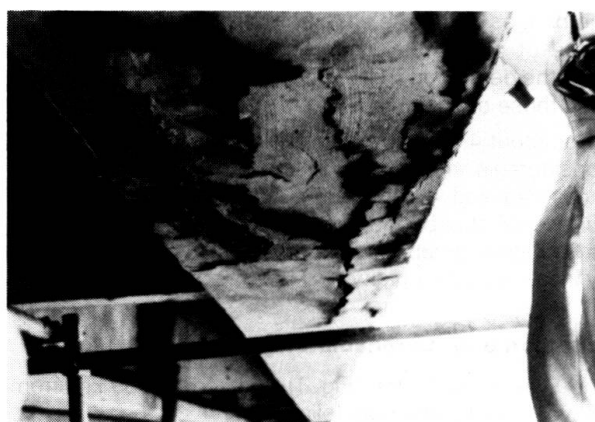
Fig. 3 Crack at lower flange (Oyataroh Bridge)
