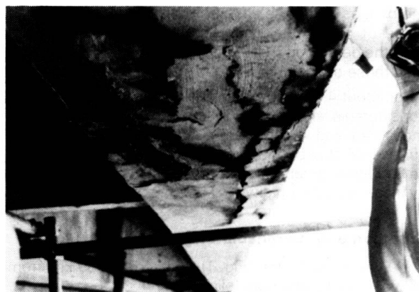
Fig. 3 Crack at lower flange (Oyataroh Bridge)
