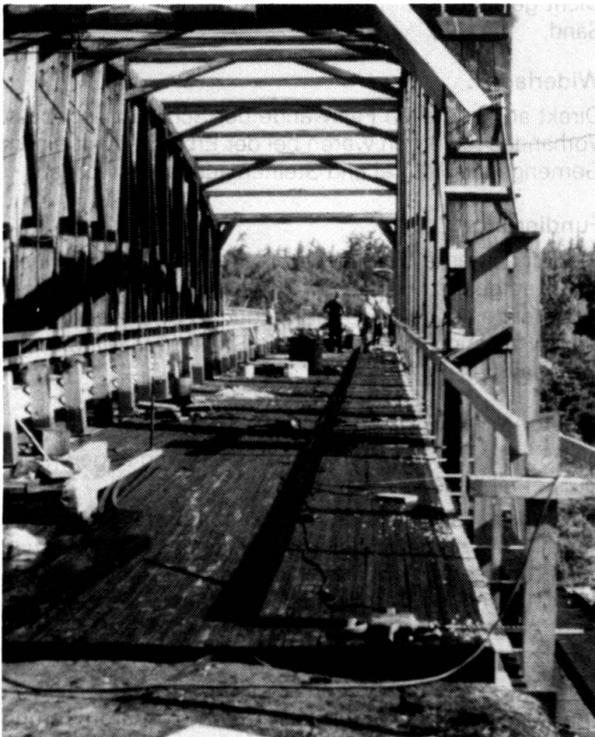
Fig. 3 Placing prestressed wood deck
