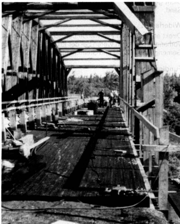
Fig. 3 Placing prestressed wood deck
