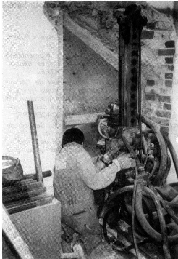
*Fig. 2 Through excavations in the supportive brick walls holes were sunk vertically through the basement walls.*
