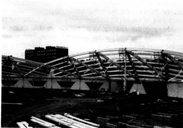
Erection of the dome
