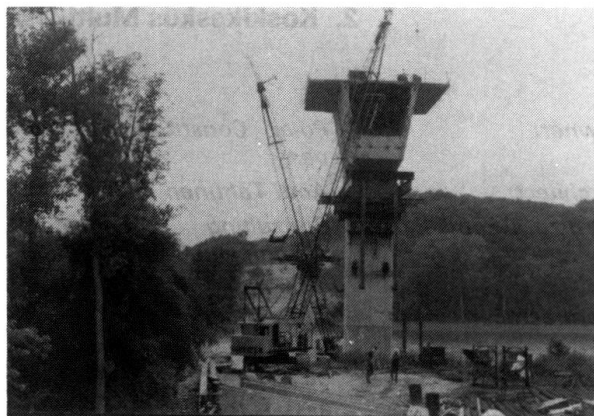
Fig. 5: Free cantilevering construction in progress
