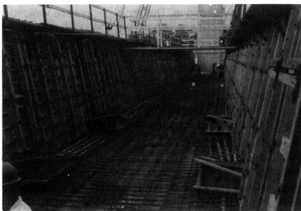
Fig. 4: After placing of inner web formwork
