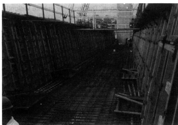
Fig. 4: After placing of inner web formwork
