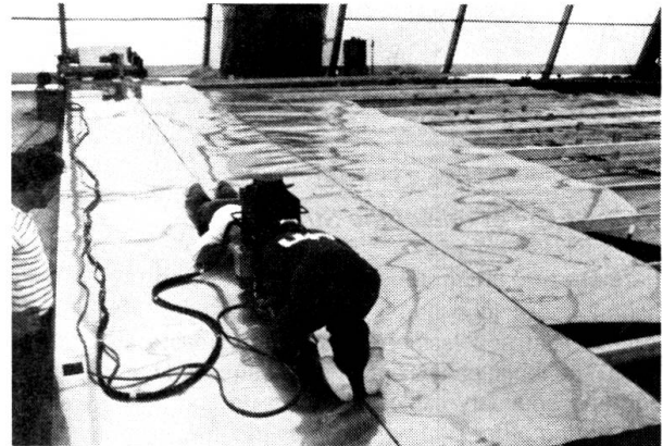
Fig. 2: Welding of the Membrane
