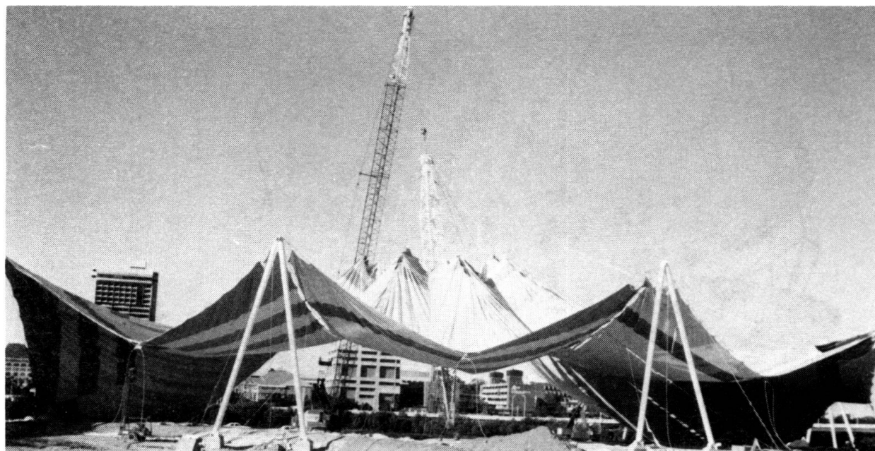
Fig. 3 Raising the membrane for one of the structures
