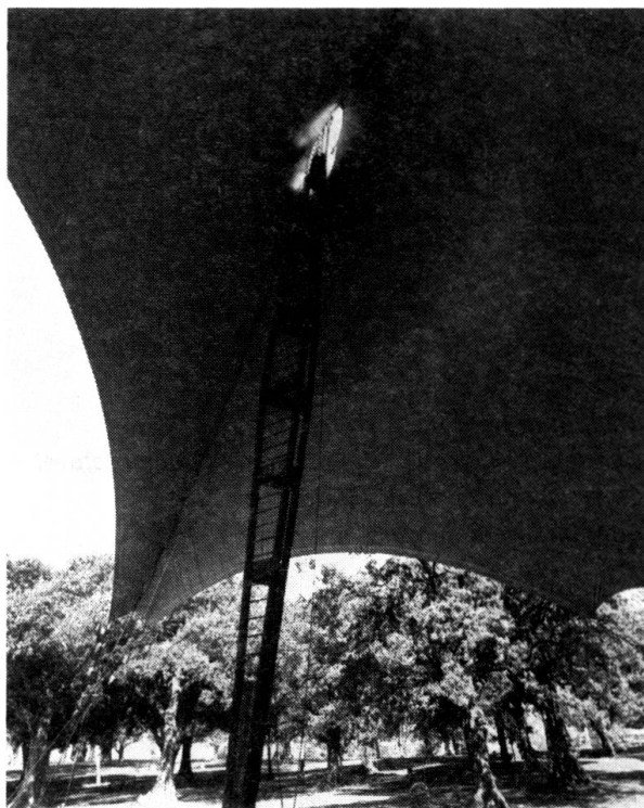
Fig. 4 Underside view showing mast, membrane corner and fabric pattern
