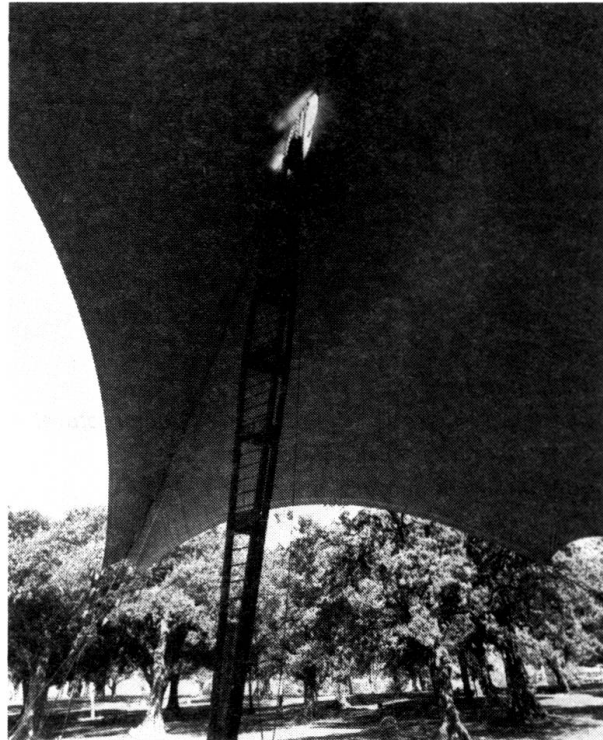
Fig. 4 Underside view showing mast, membrane corner and fabric pattern
