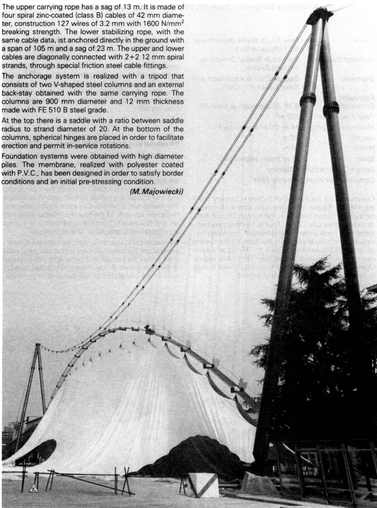
Fig. 3 Main rope truss and membrane during erection
