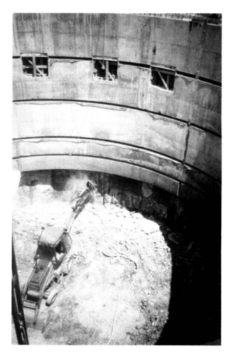
Preparation of slurry wall for casting of liner wall
