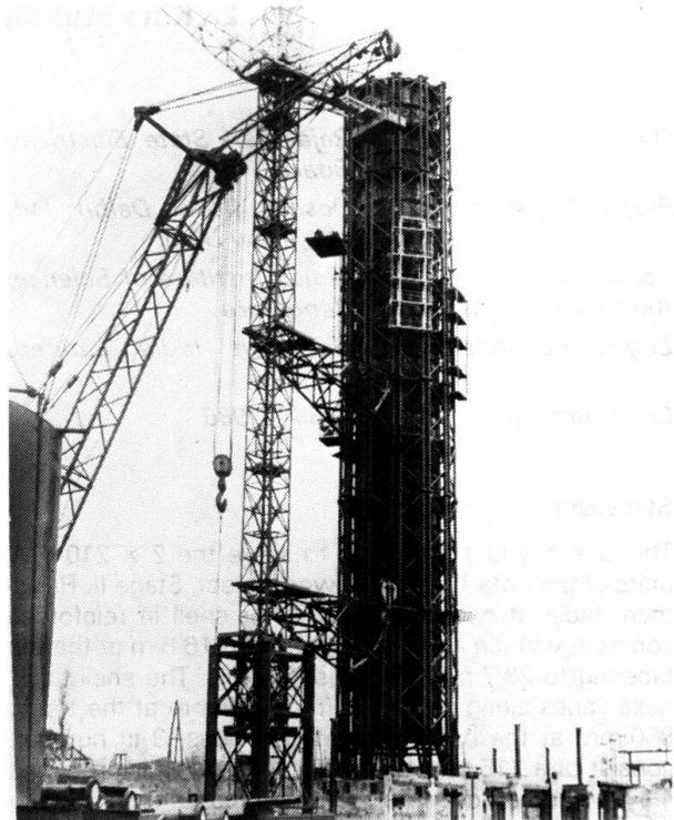
Fig. 3 Beginning of the metal tower erection
