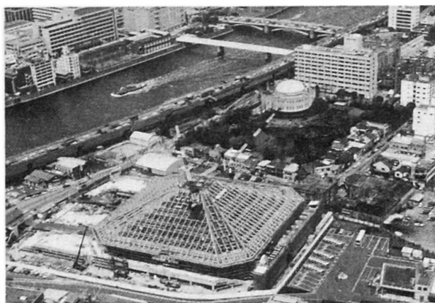
Space frame under construction
