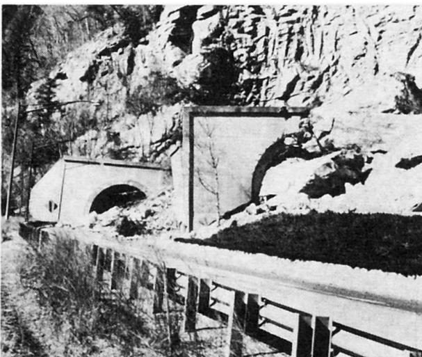
Fig. 1 Tunnel portal destroyed by rock slide
