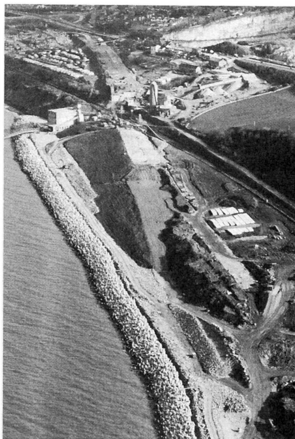
Fig. 3 Aerial view of foreshore on completion of placing Dolos units
