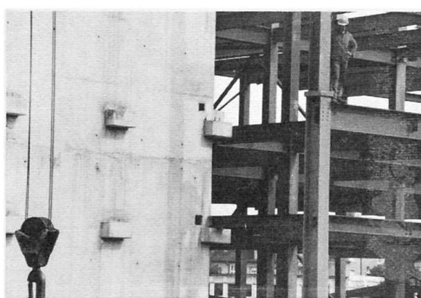
Fig. 5 Staircase with brackets
