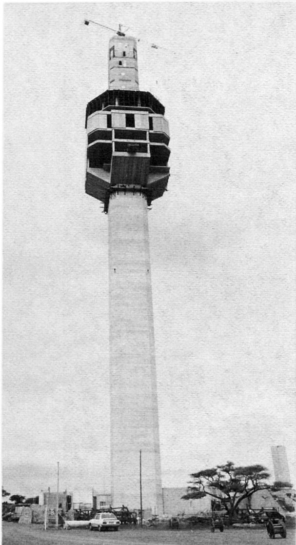
The shaft of the tower is a basic 9 m square shape with chamfered corners providing a seven-cell structure to accommodate a lift shaft and lobby, stairwell and four service ducts at each corner. At the 75 m level is the base of the major cantilever structure which supports the technical floors. Above that are the four cantilevered octagonal antennae platforms and the VHF room.
