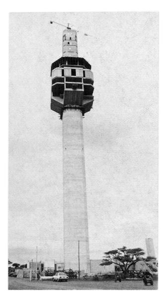
The shaft of the tower is a basic 9 m square shape with chamfered corners providing a seven-cell structure to accomodate a lift shaft and lobby, stairwell and four service ducts at each corner. At the 75 m level is the base of the major cantilever structure which supports the technical floors. Above that are the four cantilevered octagonal antennae platforms and the VHF room.
