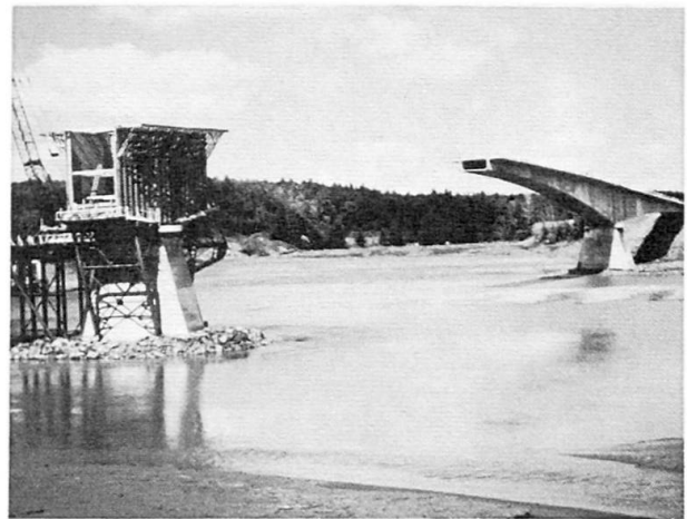
Fig. 2 West pier table at low tide
