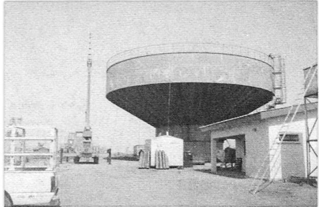
*Water tower reservoir ready. The shaft is erected by jacking up method*
