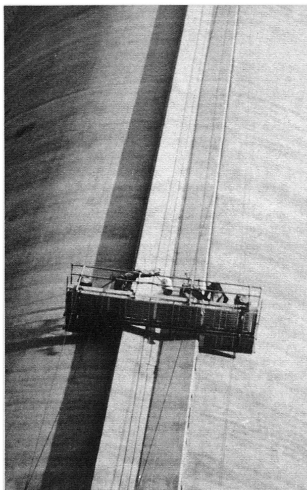
Fig. 5 VSL crew scaffold doing post-tensioning operations
