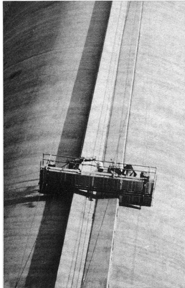
*Fig. 5 VSL crew scaffold doing post-tensioning operations*
