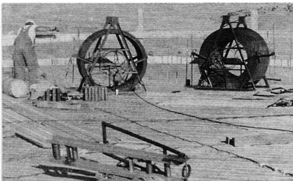
*Fig. 4 Packs of strand on the silo roof*
