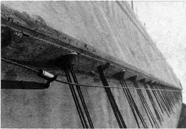
*Fig. 3 Buttress with anchorages VSL type B*
