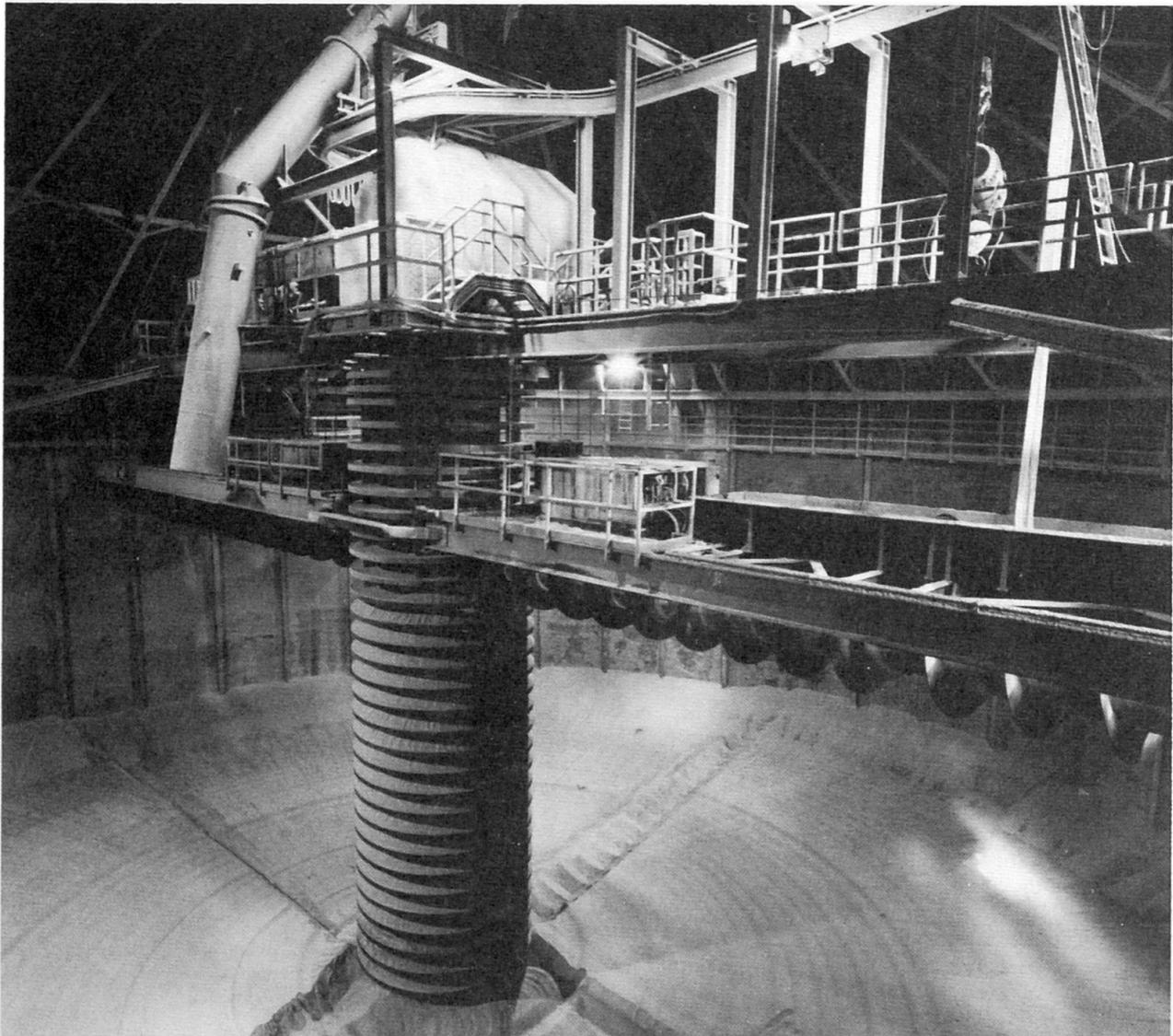
Fig. 3 Bridge crane and reclaimer installed in silo
