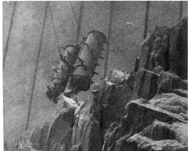
**Fig. 1** Potash hanging up on silo wall
