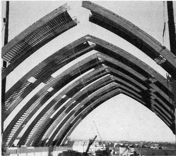
Fig. 2 *Glulam arches form centre barrel section*
