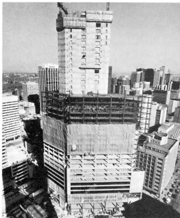
(G.A. Culham) Fig. 3 Tower under construction
