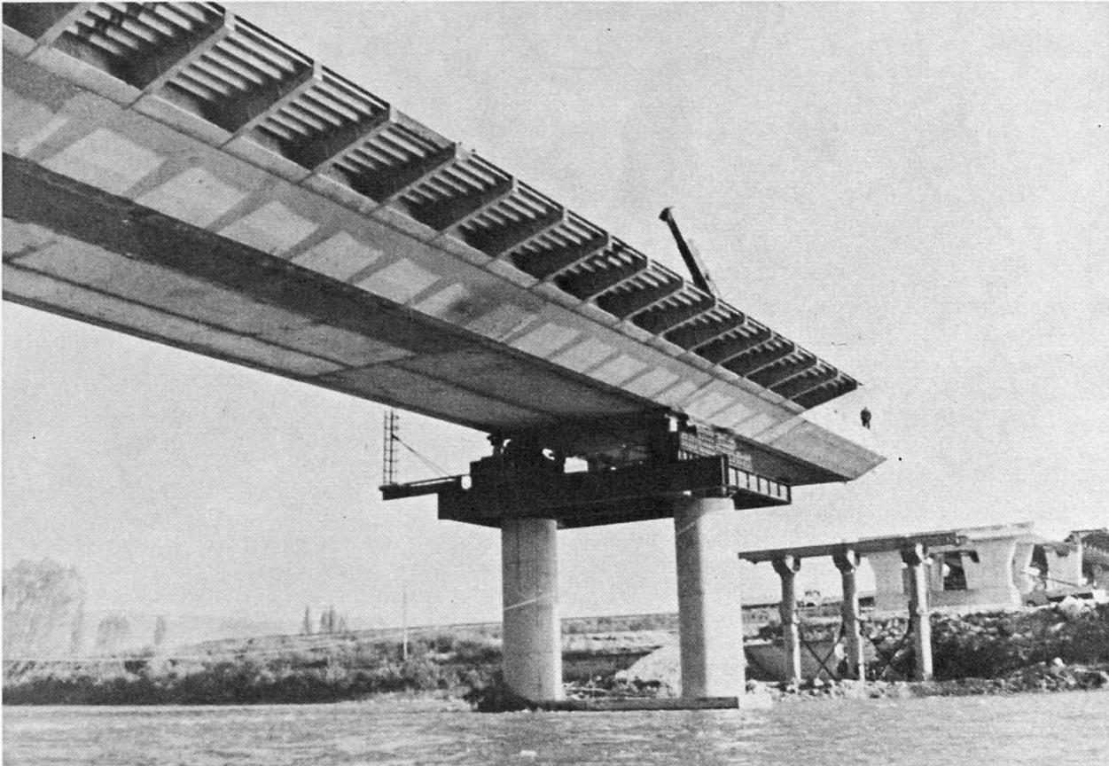
*Fig. 2 The positioning of the main beam*
