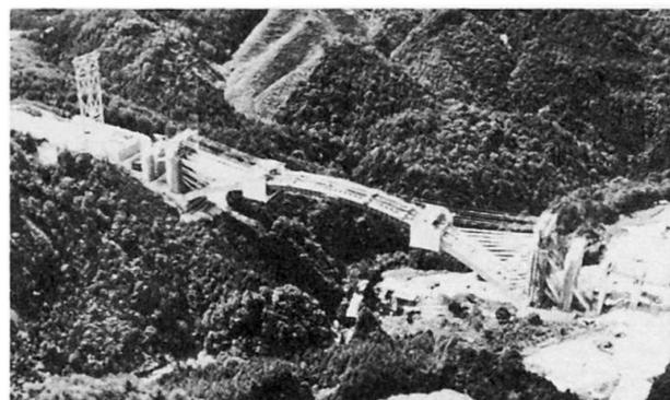
Fig. 2 Construction over a steel girder arch
