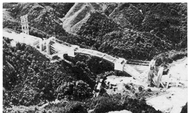
Fig. 2 Construction over a steel girder arch
