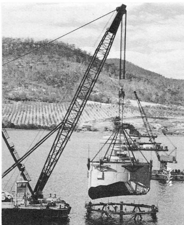
Fig. 4 Lowering first segment Pier 2 Cofferdam
