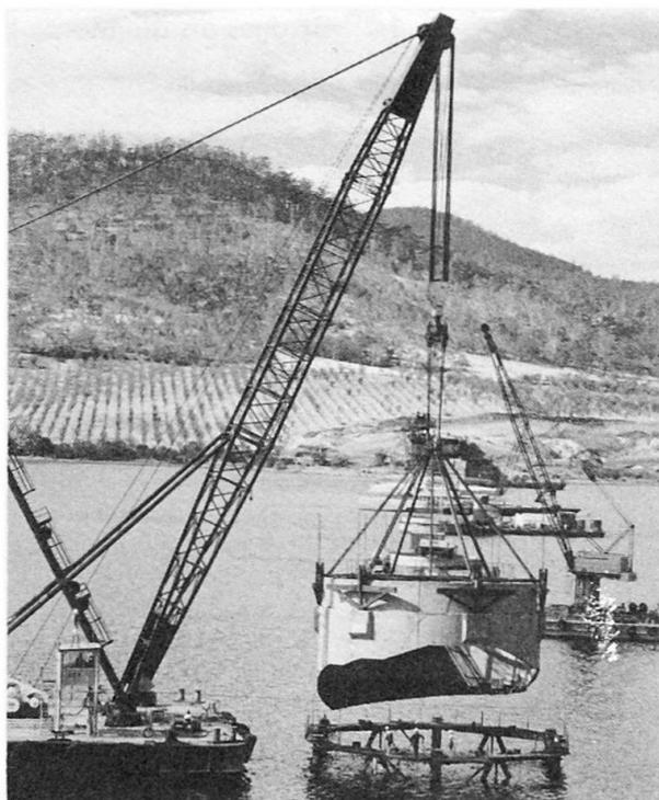
**Fig. 4 Lowering first segment Pier 2 Cofferdam**
