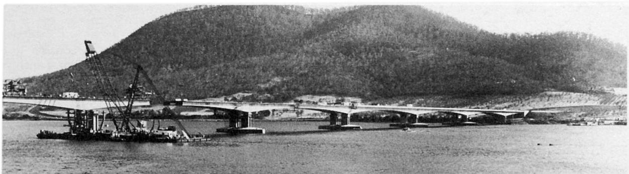
**Fig. 5 Cantilever erection of deck**
