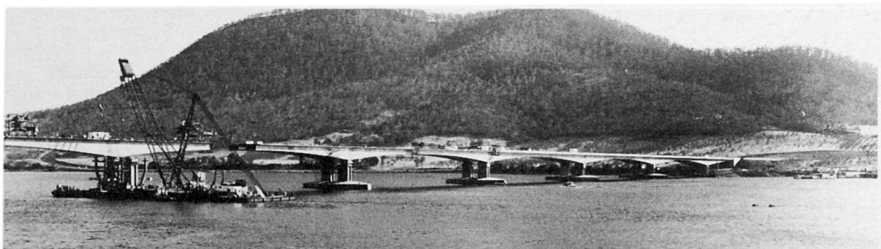
Fig. 5 Cantilever erection of deck
