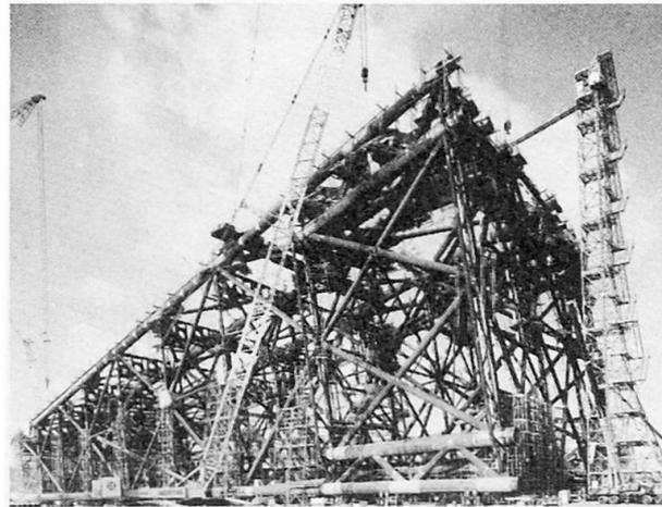
**Fig. 4** *The 15,000 ton Iwaki platform jacket under construction*
