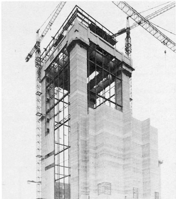
**Fig. 4** Prestressed reinforced concrete girder grill in its final position. Construction of the rigid connection of the girder grill and the pylons. Installation of cladding between the pylons.
