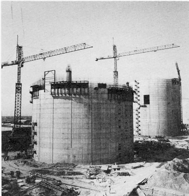
**Fig 2** General view showing construction of containment walls
