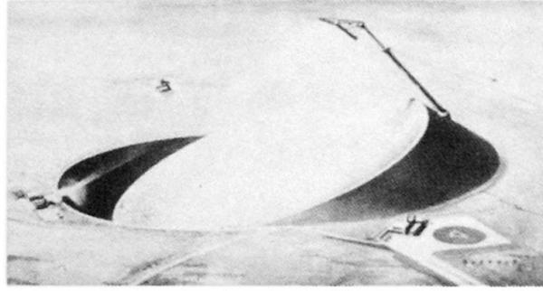
Fixed membrane mirrors of say 80 meters diameter with thermal power of 4500 kW or electrical 750 kW.
