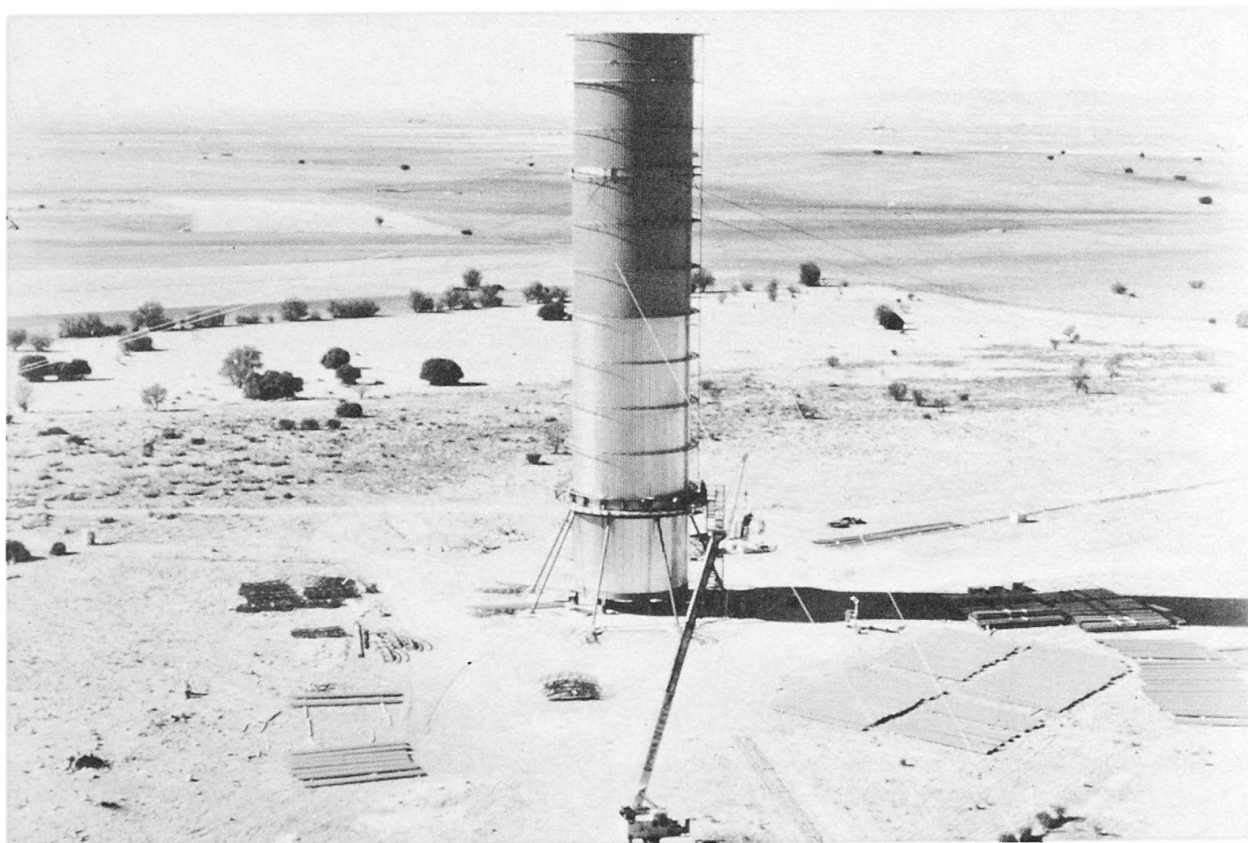
Fig. 15: The erection of the chimney by incremental lifting
