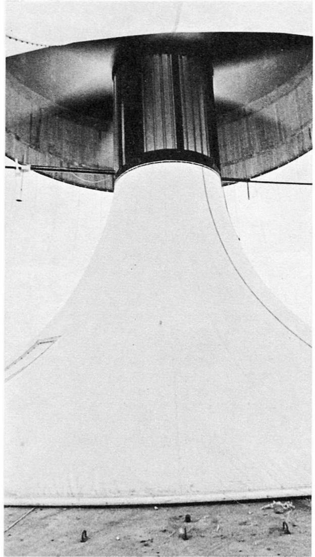
Fig. 21: The funnel providing a smooth transition from the collector's horizontal airflow into the chimney's updraft
