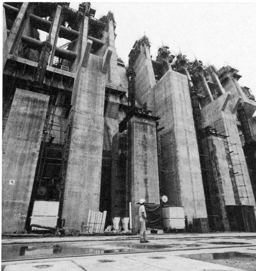
Hollow gravity dam
