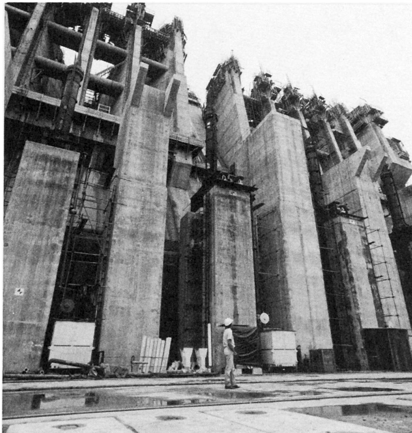
Hollow gravity dam
