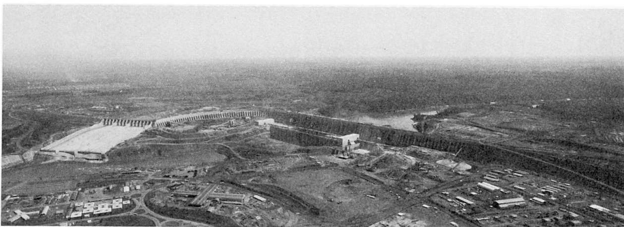
General view of Itaipu dam in final construction phase
