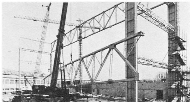
Fig. 2 Erection of steel trusses
