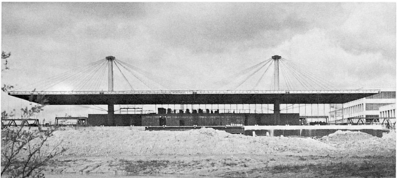
**Fig. 2** *Roof under construction showing cable system*
