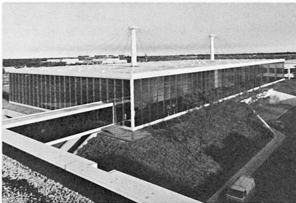
**Fig. 1** *The suspended roof system for Baxter Laboratories Dining Hall*
