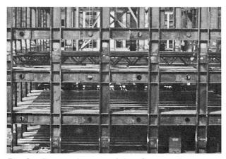
Fig. 6 Beam-column modules after erection
