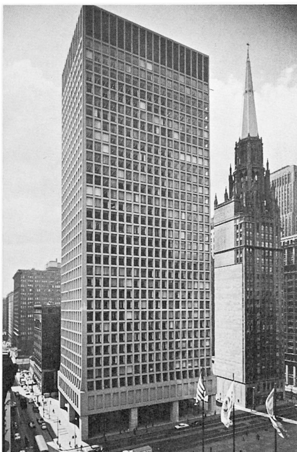
Fig. 1 Brunswick Building, Chicago, Illinois
