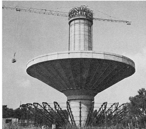
Fig. 4. Shell during lifting
