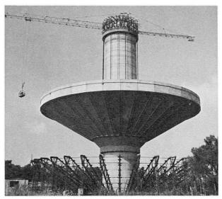
Fig. 4. Shell during lifting
