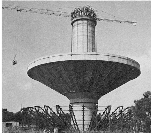
**Fig. 4. Shell during lifting**
