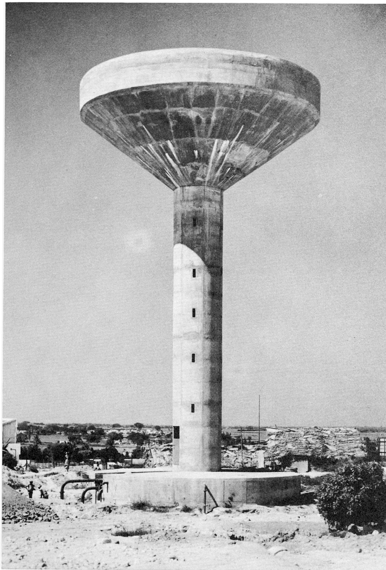
Water tank with ferro-cement suspended shell roof near Bangalore
