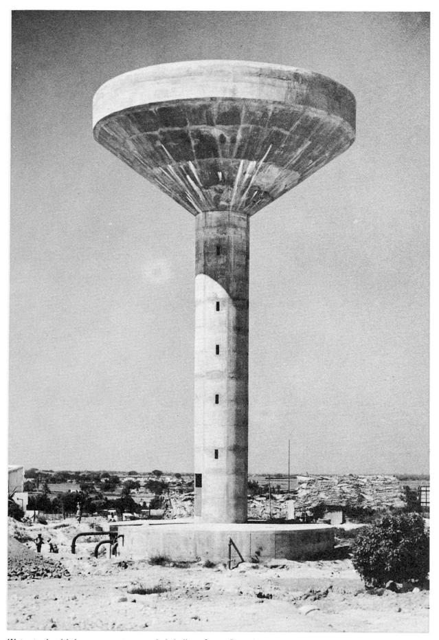
Water tank with terro-cement suspended shell roof near Bangalore
