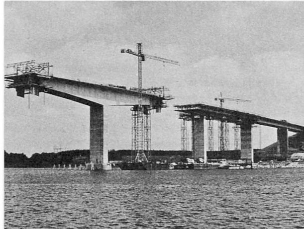
*Casting of approach span and cantilever construction symmetrically from main pier*
