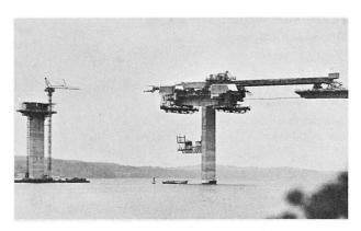
105 m launching steel girders were used for the cantilevering operation
