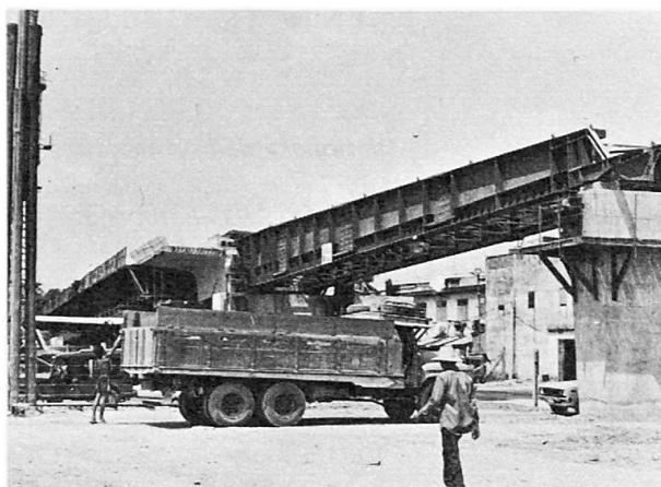
Approach spans during construction
