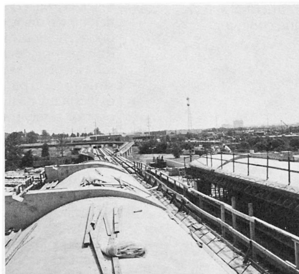
Fig. 5 Upper tier canopy after concreting
