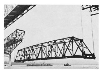
Fig. 4 South bridge. Suspended span (152.5 m) free of barges being hoisted by block and tackle into final position
