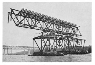
Fig. 3 South bridge. Off-site truss erected on barges being moved upstream for final erection in structure
