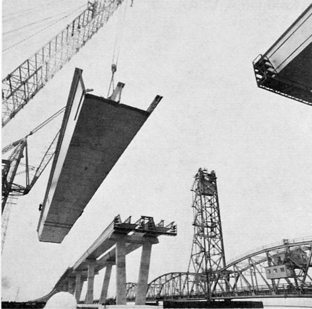
*Fig. 2 Lifting of a trapezoidal steel box girder*
