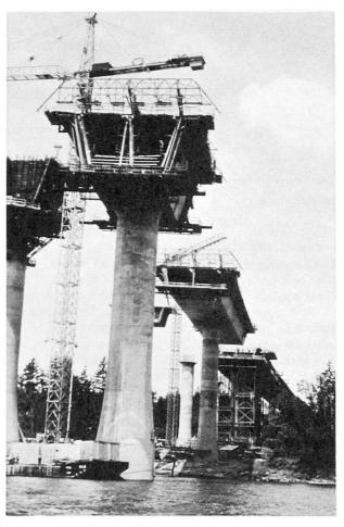
Fig. 3 Cast-in-place falsework Cast-in-place cantilever
