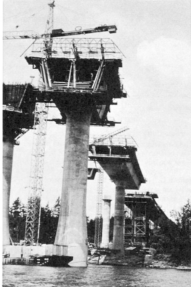
Fig. 3 Cast-in-place falsework
