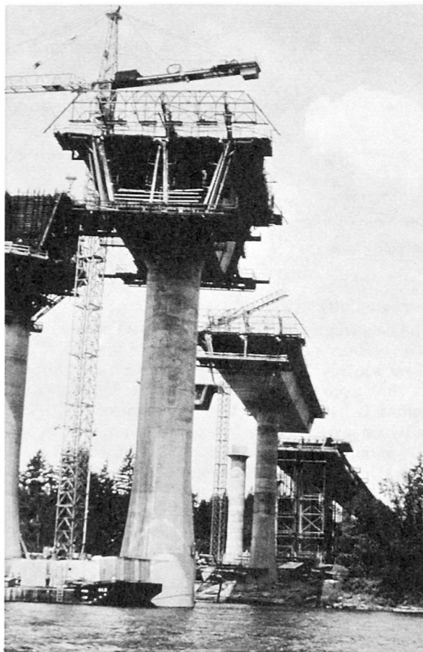
Fig. 3 Cast-in-place falsework Cast-in-place cantilever
