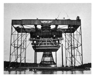
Fig. 2 Pile cap form
