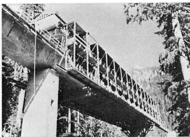
Fig. 1 Movable truss scaffold moves from pier to pier across the valley of Denny Creek, leaving behind the bottom and sides of post-tensioned box girder that will support the forms for casting the top and deck of the bridge superstructure.
