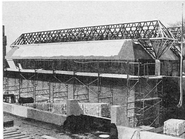
Fig. 4 Steel girder in the gymnasium block
