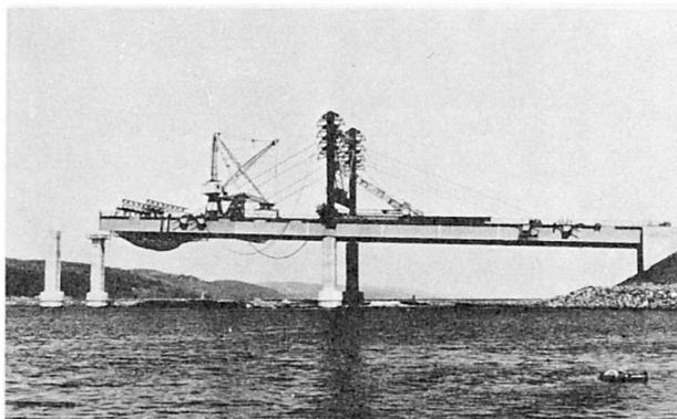
Fig. 4 Cantilevered erection of approach spans showing temporary towers and cables, and other erection equipment
