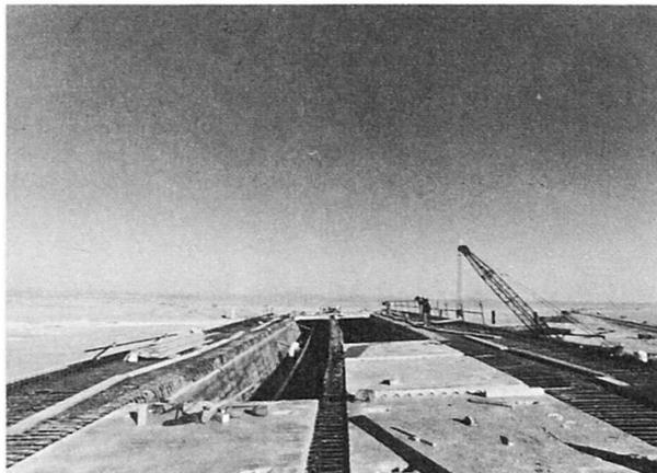
Fig. 4 Placing of the precast deck slab elements after concreting bottom slab and webs and applying a partial prestress
