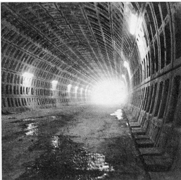
Tunnel driving commenced in January 1979. During the first year of driving an average production of 18 rings per week was achieved representing 21.6 m complete with road deck. During a period from August 1979 until the end of February 1980, an average advance of 30 m per week was maintained.
