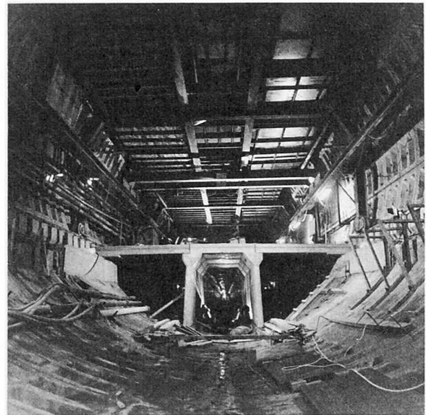
The road deck is of P.C. concrete units (the central culvert unit weighing 12 tonnes) placed by a gantry crane running under the shield trailers.
